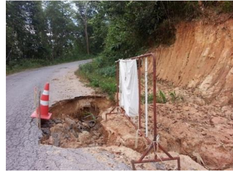
Erosion near Pumuen village, caused by relatively new impervious road surface.
