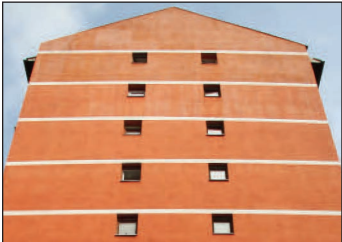
This is the same apartment building as above, in 2009. The front side remains heavily damaged. Many homes and other buildings in Sarajevo have been either repaired or built, especially since 2007.
