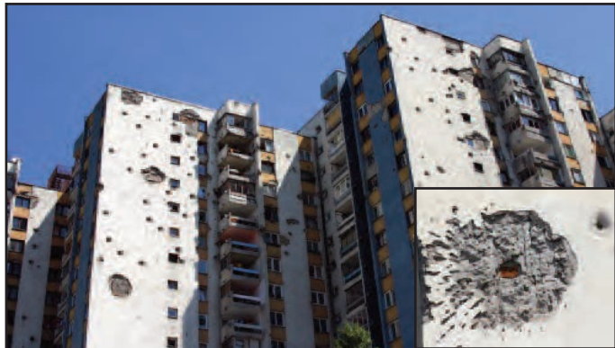
This is an apartment complex pockmarked with holes left by artillery shells – remnants of mass destruction that the world watched from afar.
